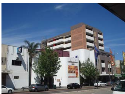
Photo 1 Existing Castellorizian Club, with redevelopment of No. 450-458 Anzac Parade substantially completed
