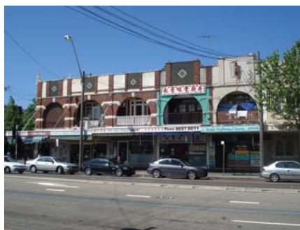
O:\Business Papers\MINUTES, AGENDAS\2007\Minutes_Agendas\Ordinary\11-27 Business Paper-no frp.doc projecting wall signs have been installed on the ITEM 8.4 building. The above signs have a height of less than 5m.
