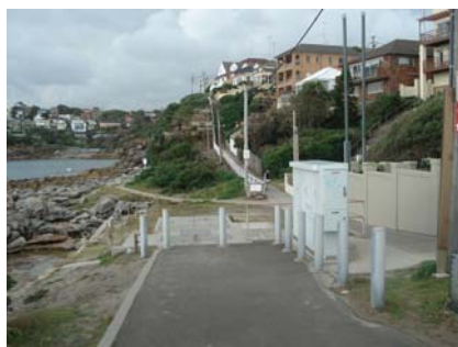
Photo 4 Cliffbrook Parade and pump-out station
